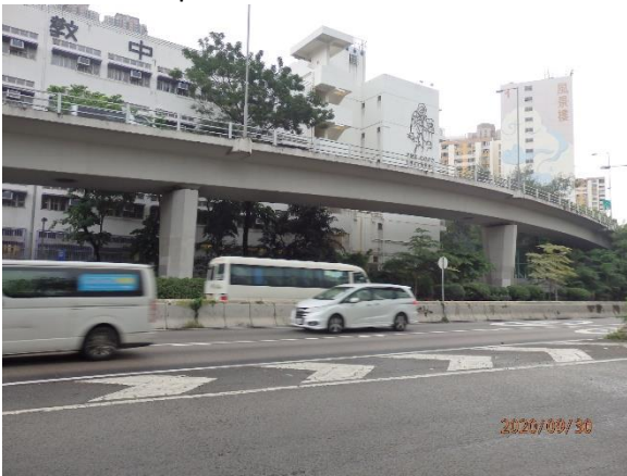
Photo 21. Kwai Chung Road
