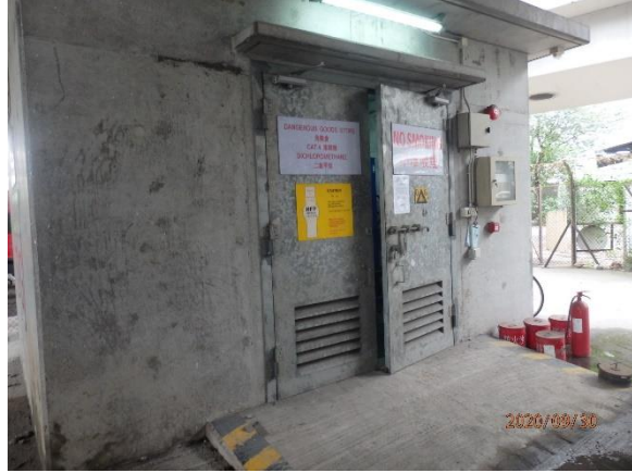
Photo 2. Store for Dichloromethane constructed in 2014
