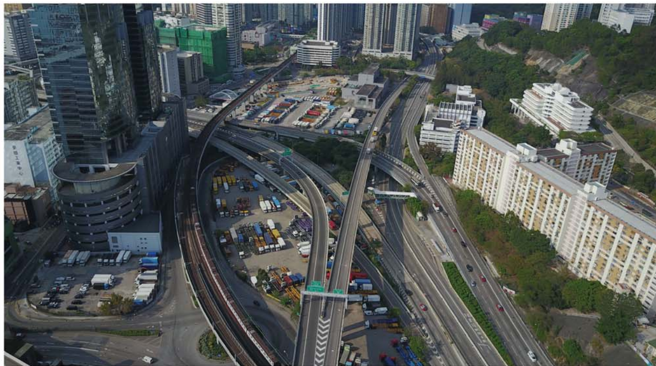
Existing Site Condition
