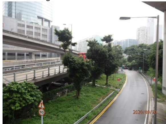
Photo 24. Container Port Road South
