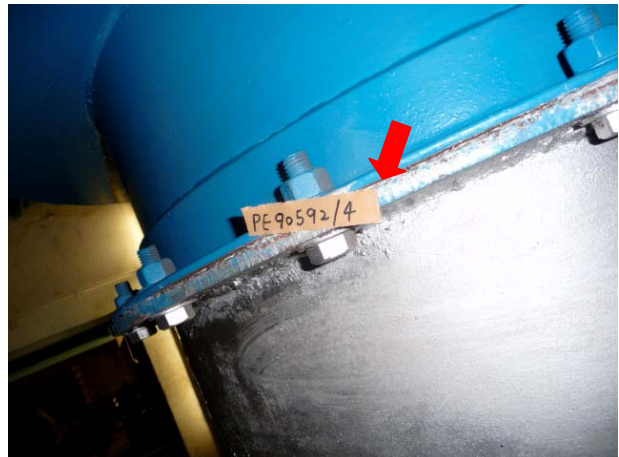
Photo 4. Chimney Gasket (PE90592/4) sampled at Chimney of Incinerator 2 was confirmed as Non-ACM.
