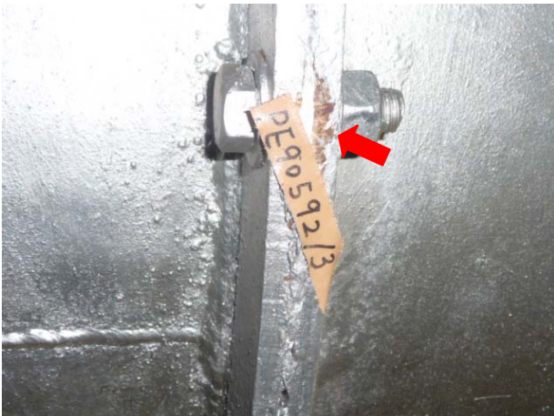
Photo 3. Chimney Gasket (PE90592/3) sampled at Chimney of Incinerator 1 was confirmed as Non-ACM.
