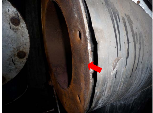
Photo 8. Metal Chimney with no gasket, photo taken at the outside of Incinerator Room.
