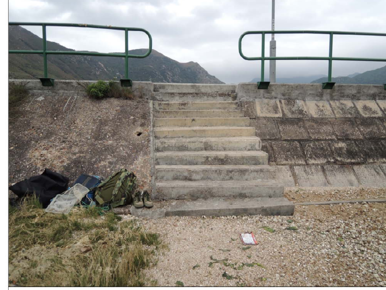
⑧ EXISTING STAIRCASE TO BE REMOVED AND REINSTATED AFTER CONSTRUCTION 現有樓梯臨時清除並於竣工後恢復原狀
