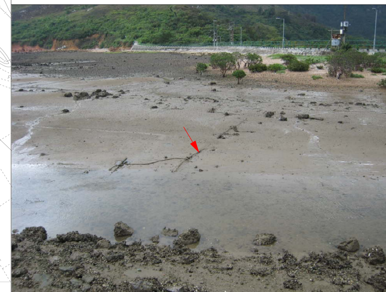
⑥ PARTLY EXPOSED EXISTING CABLE 現有露出電纜
