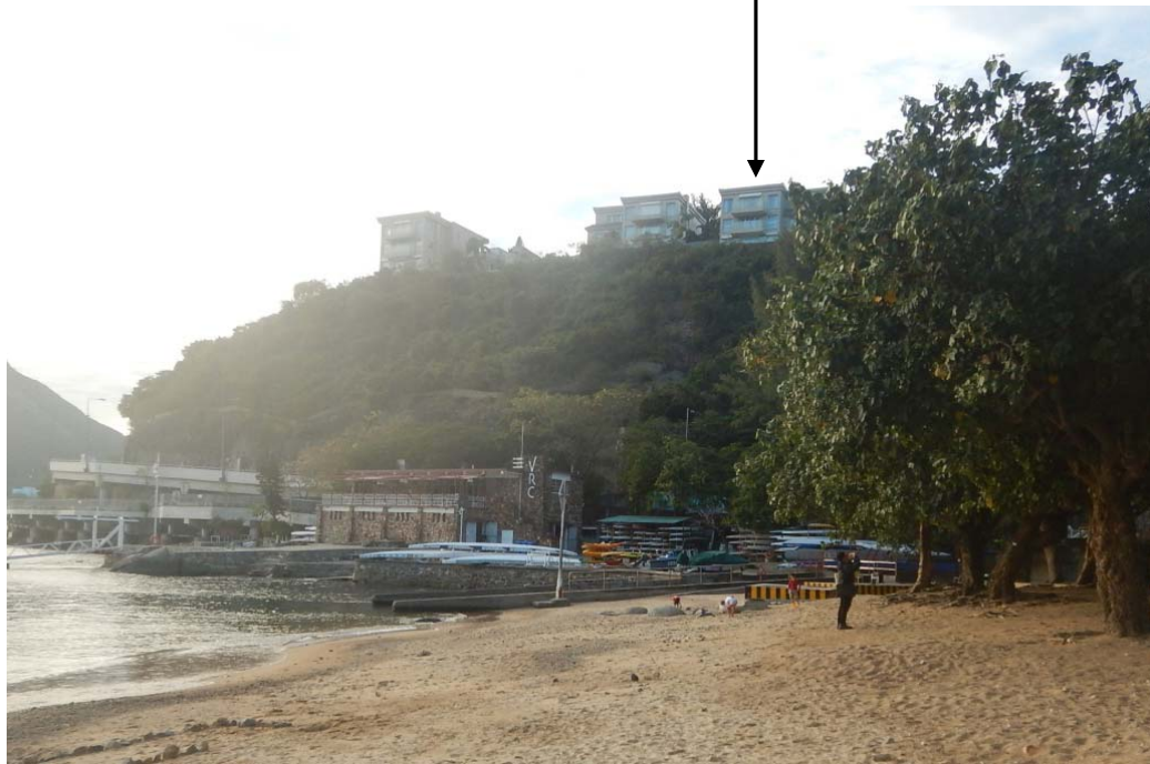
House 3, Deep Water Bay Road No. 72 (N1) 深水灣道72號, 3号屋 (N1)
