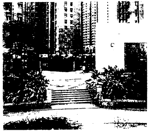
Photograph 2- High-rise Residential Area Residential space and entrance at Kam Lung Court
