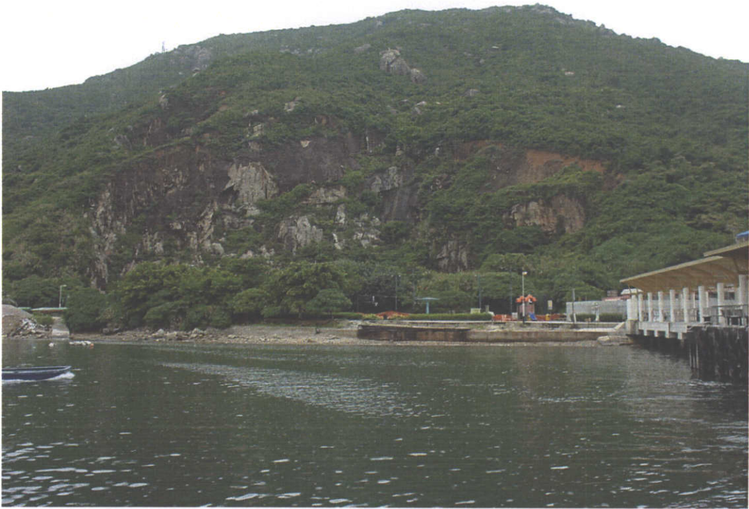
Plate 1: General view of the project site
