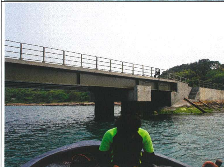
Plate 30. The completed product. A new pier at Tung Ping Chau.
