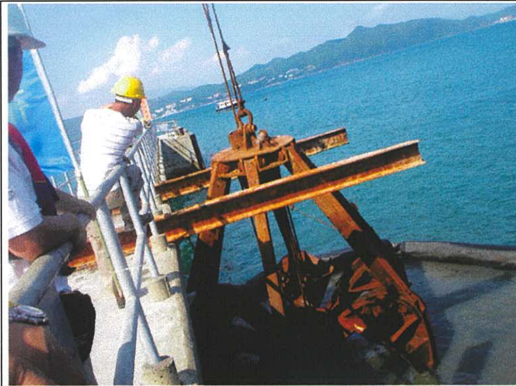
Plate 19. Accurate grabbing within metres of a coral area. This work was supervised from the surface in-water. No coral damage resulted. A similar technique had been applied during the Pak A project.
