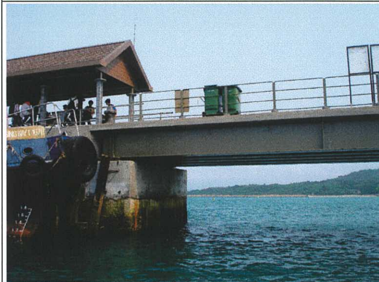
Plate 29. The far end of the new pier.
