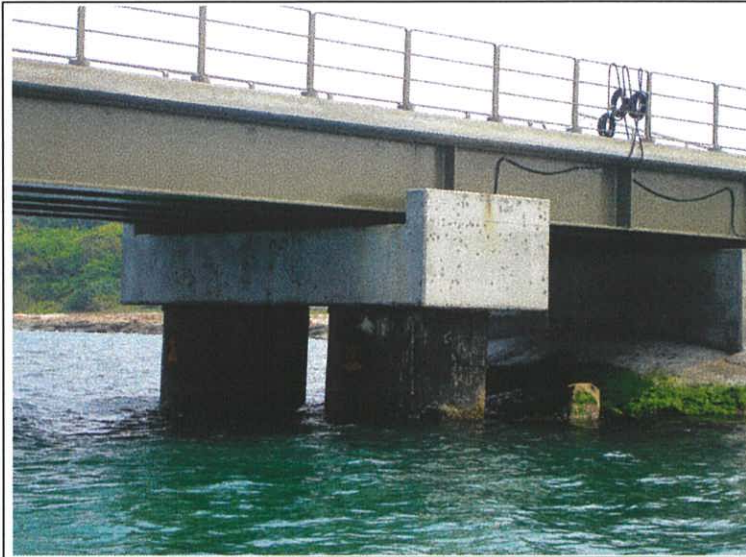
Plate 28. A closer view of the new pier.
