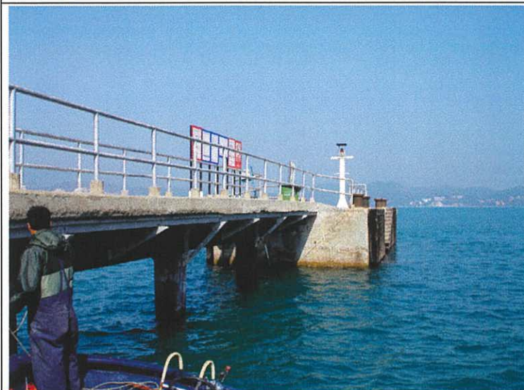
Plate 2. The old pier before the renovation works began.
