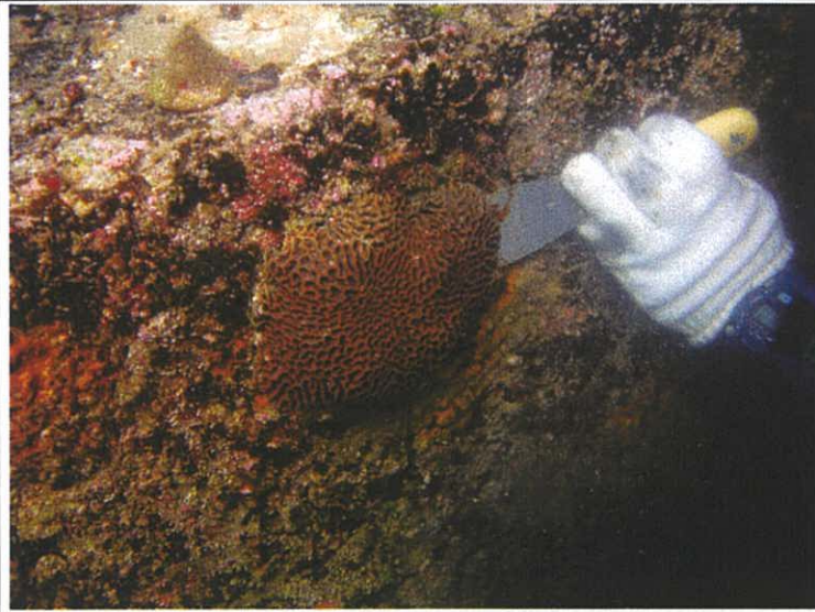
Plate 4. Removing a small encrusting coral from the pier foundation before the works started.
