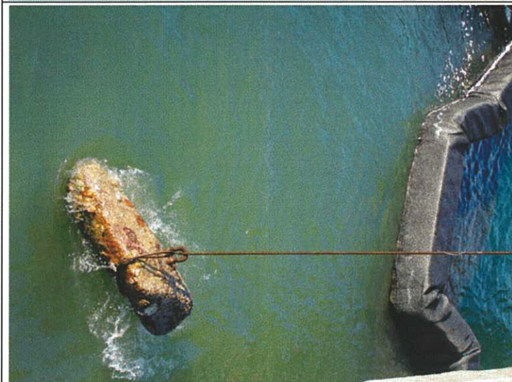
Plate 12. A foundation rock being lifted out.
