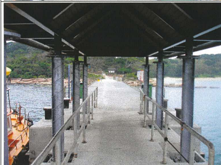
Plate 24. A photograph along the new pier. Only some of the railings had not been installed.
