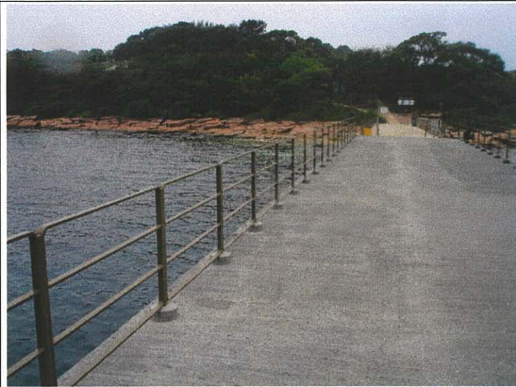
Plate 25. Along the new pier. (March 2007)
