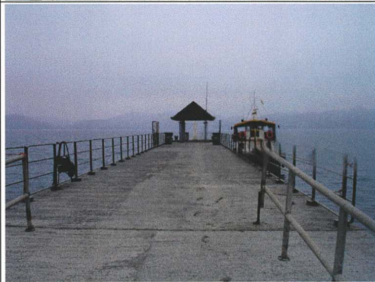
Plate 26. Looking towards the end of the new pier. (March 2007)
