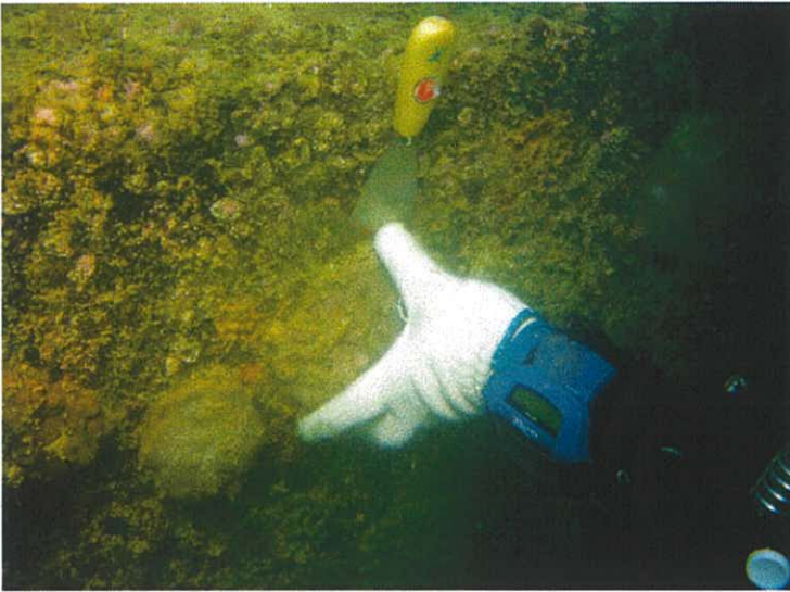
Plate 7. Another nearby colony being detached from the pier footing.
