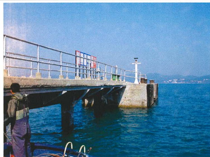
Plate 2. A view of the mooring end of the pier.
