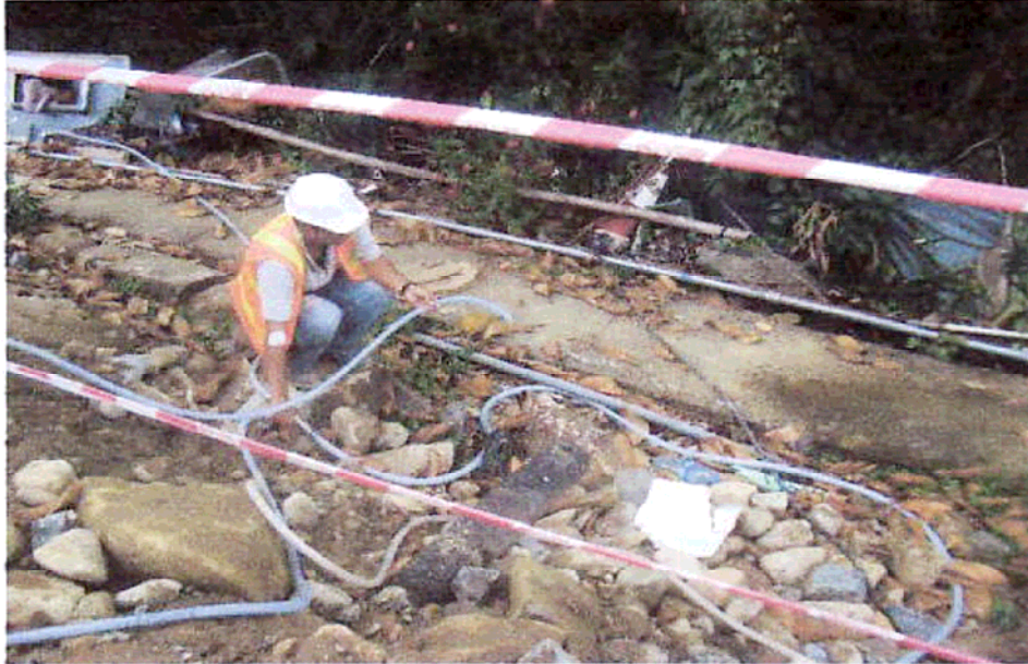
(Fig 2) High jet water sprayer was provided for washing vehicles, photo taken on 3 rd December 2008
