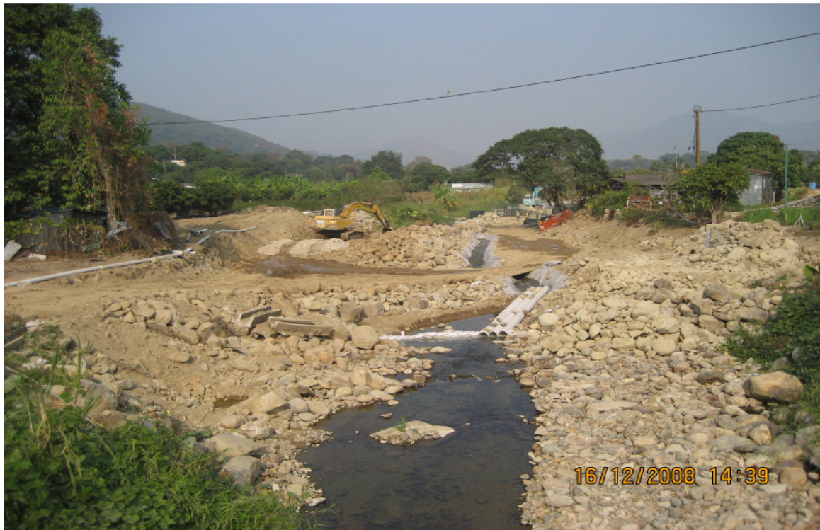
Fig.5 Bunds without coverage of geo-textile at ch.0 of LTR
