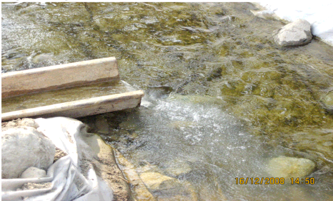
Fig.2 Discharge from the branch to the river channel of LTR (at ch.250~300)
