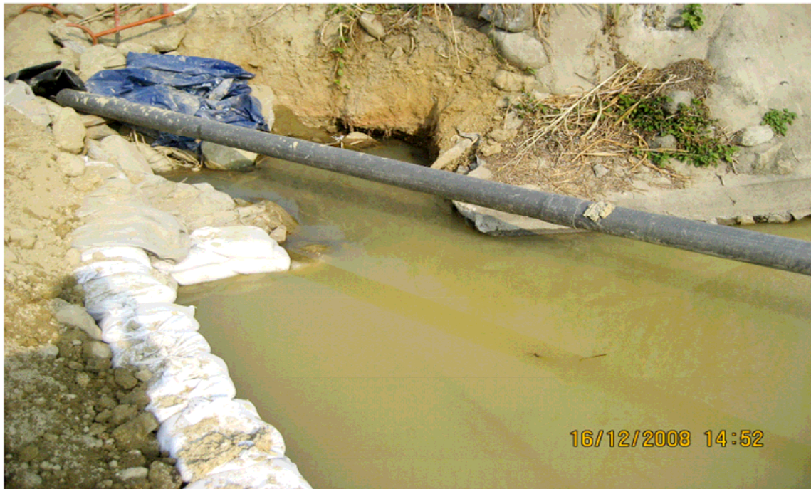
Fig.1 Site water was directly discharged to the branch of LTR (at ch.250~300)
