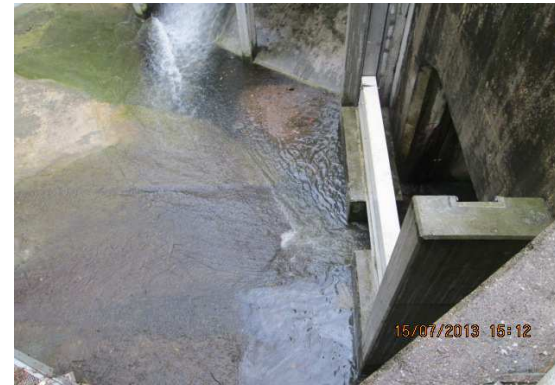
Photographic record for exceedance of Turbidity recorded at Sik Sik Yuen Ho Fung College (I-1) on 15-Jul-13
