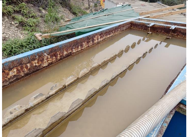
Silt Removal Facility in Portion A
