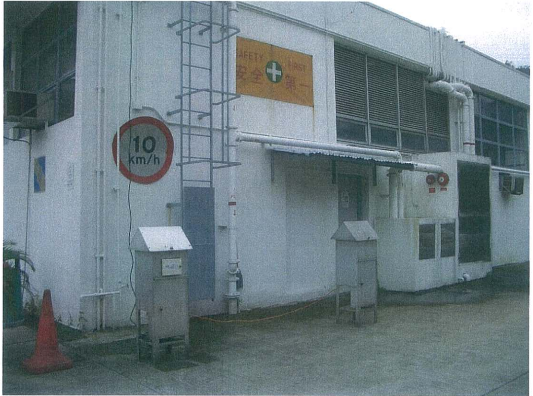
AM1 – Tuen Mun EMSD Servicing Vehicle Station
