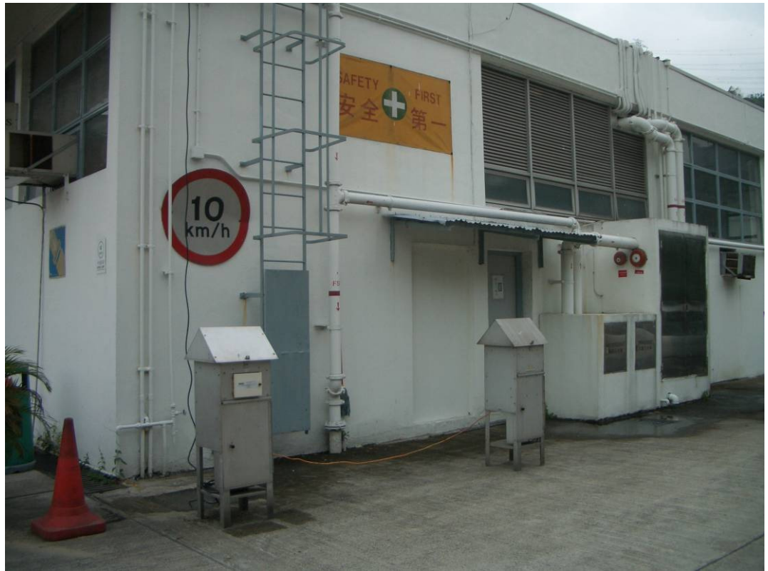
AM1 – Tuen Mun EMSD Servicing Vehicle Station
