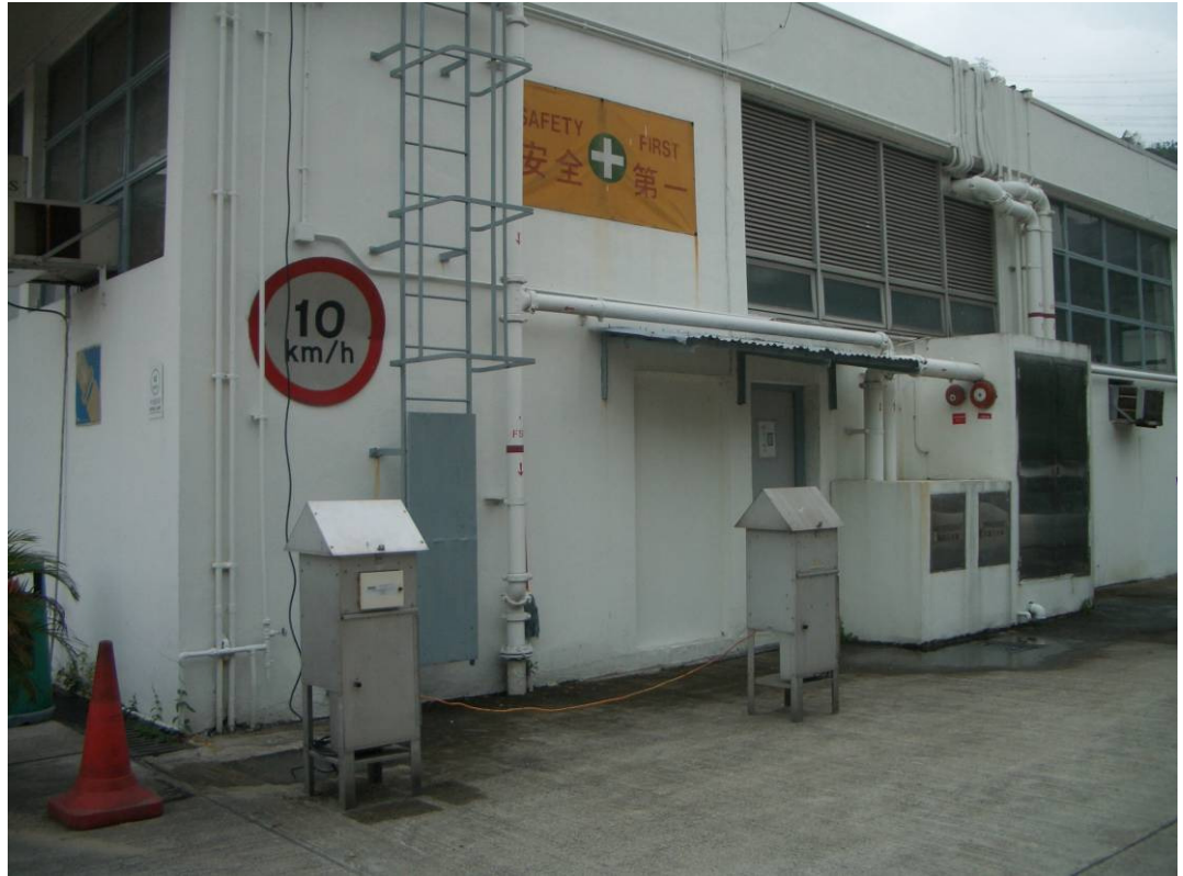
AM1 – Tuen Mun EMSD Servicing Vehicle Station
