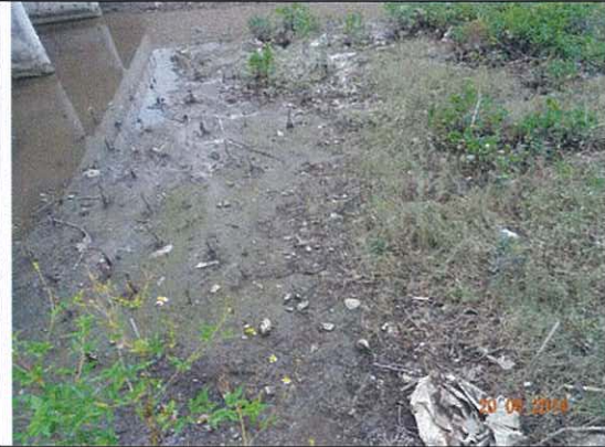
10. Current inspection : Rubbish from upstream was cleared up in this quadrante
