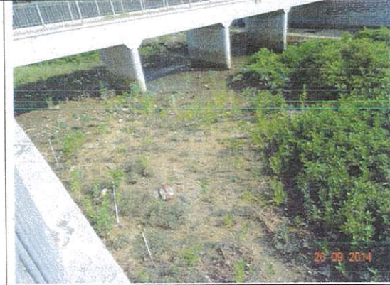
14. Current inspection: No significant change
