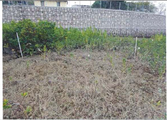
18. Current inspection: No significant change
