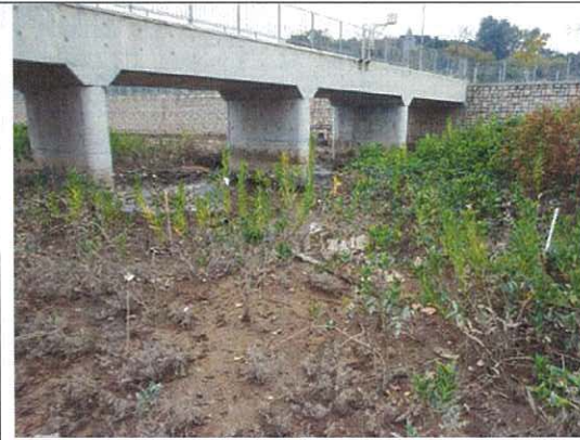
14. Current inspection: No significant change
