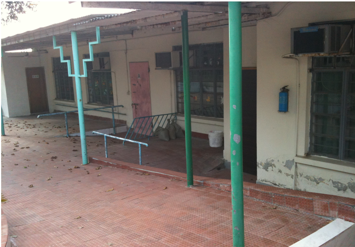
Air Quality Monitoring Station (A1) - Wing Jan Camp (Cancel)
