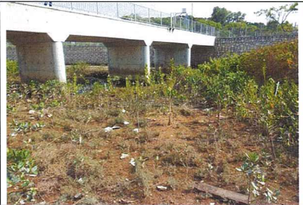
14. Last inspection in March 2015
