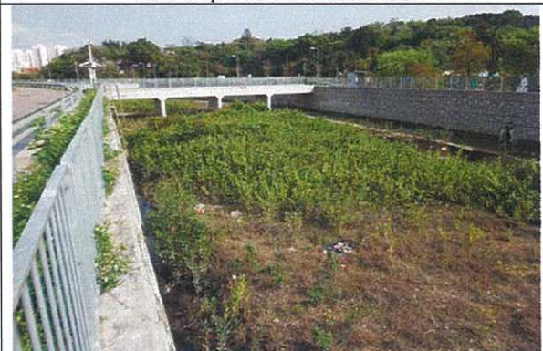
6. Last inspection in March 2015
