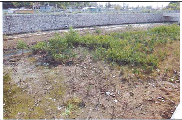
2. Last inspection in March 2015
