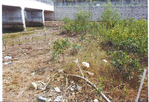
10. Last inspection in March 2015
