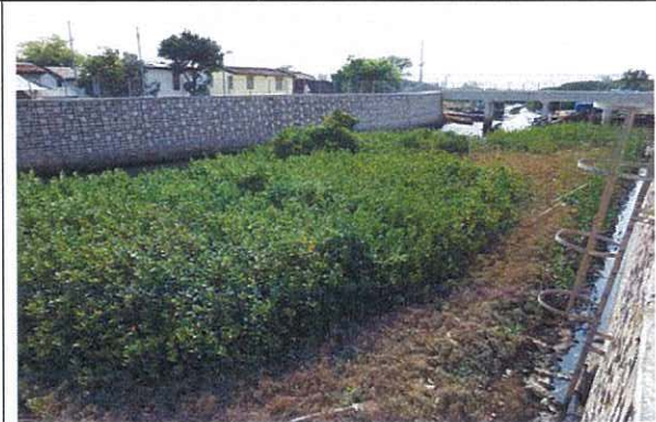
8. Last inspection in March 2015
