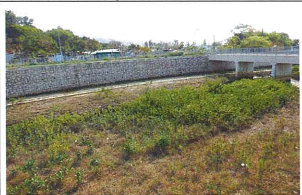
4. Last inspection in March 2015
