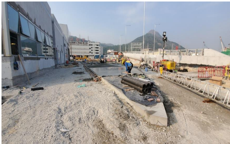
Photo 2 - Construction works at Maintenance Depot
