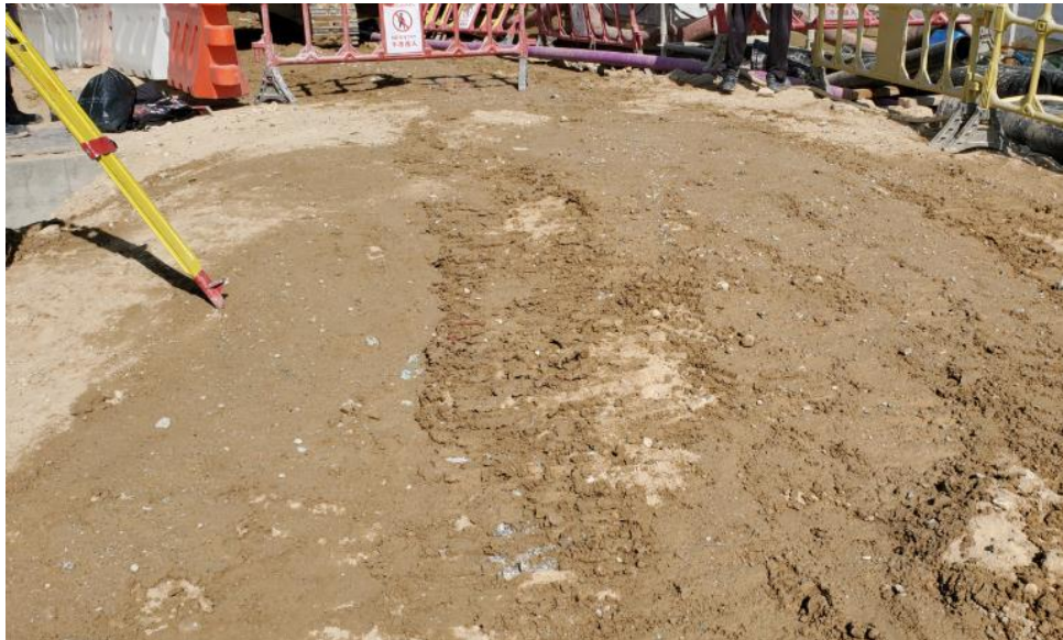
Photo 4 - Watering was applied at Administration Building
