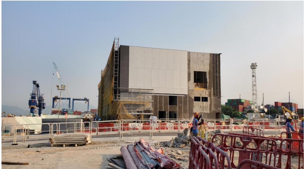
Photo 1 - Construction works at Administration Building
