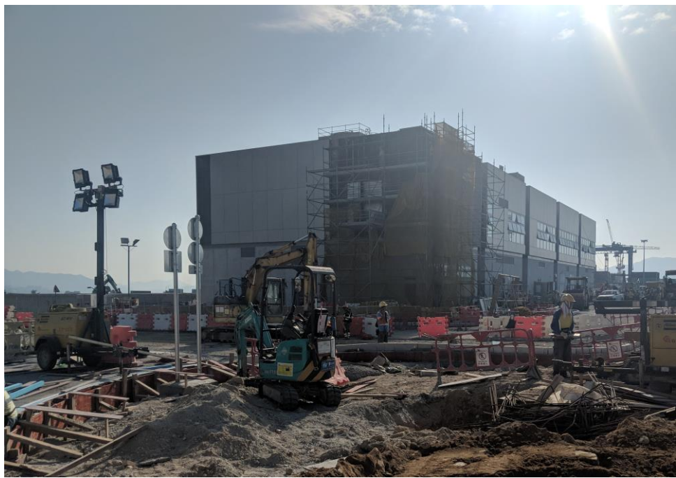
Photo 2 - Site condition at Administration Building
