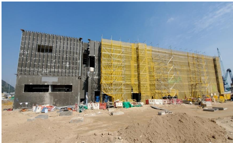
Photo 3 - Construction works at Administration Building
