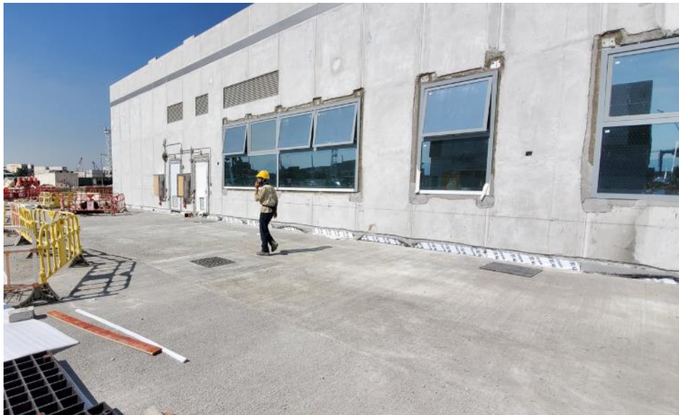
Photo 2 - Construction works at Maintenance Depot
