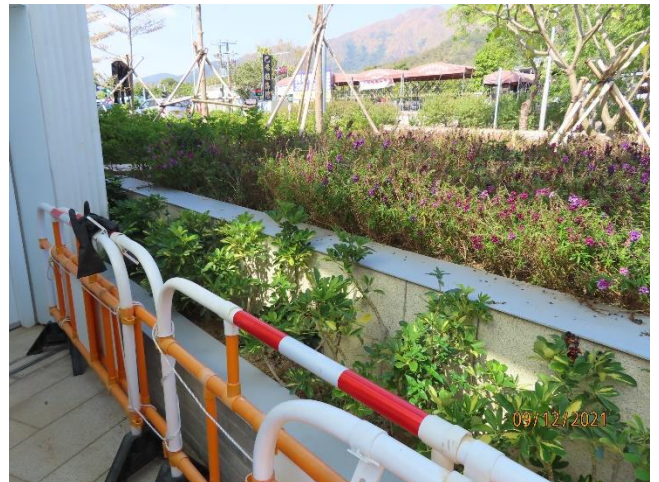
The plant near the male changing room (Planter P7) is Schefflera arboricola instead of Rhapis excelsa shown in the plan
