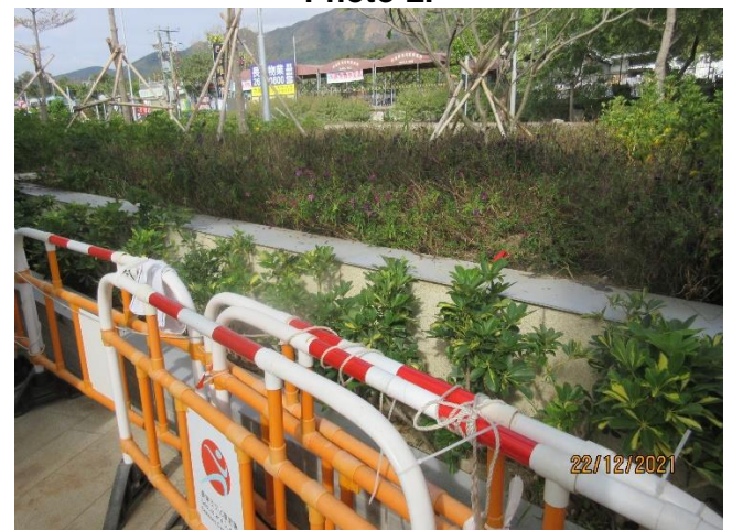
The plant near the male changing room (Planter P7) is Schefflera arboricola instead of Rhapis excelsa shown in the plan
