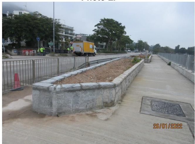
The planters at the Eastern box culvert were repaired and enlarged and the plants in the planters were removed
