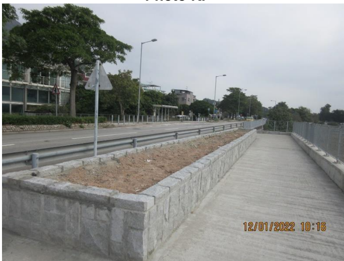
The planters at the Eastern box culvert were repaired and enlarged
