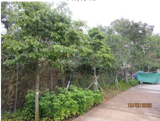
Some ties and stakes were detached at Western Box Culvert
