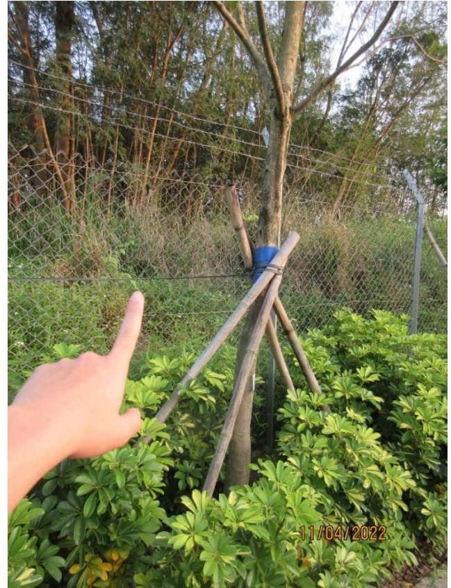
Some ties and stakes already girdled and affected the growth of the trees. Some unnecessary ties are attached between the trees
