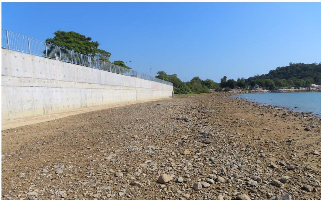
Photo 3.6 The area next to location 3
