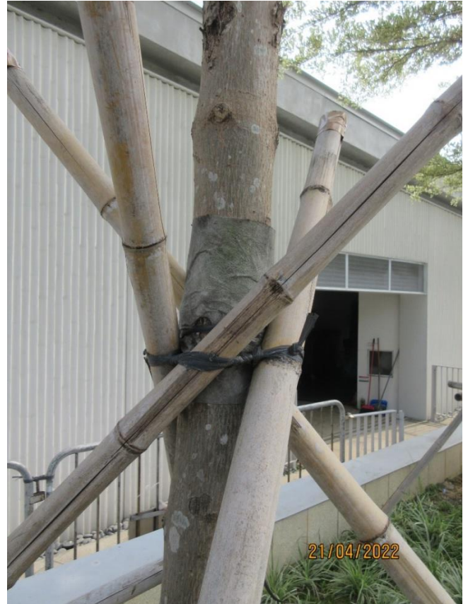
Some ties and stakes already girdled and affected the growth of the trees. Some unnecessary ties are attached between the trees
