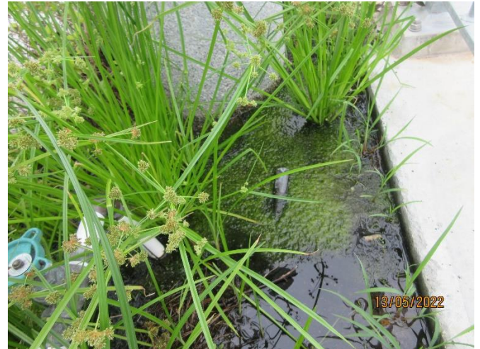
Poor soil drainage is found in one planter on the Eastern groyne.
