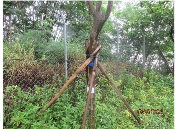
Some ties and stakes already girdled and affected the growth of the trees. Some unnecessary ties are attached between the trees.
