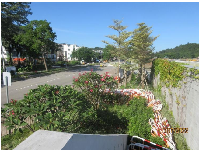
The Railing & debris damage the planters at the planter near Ting Kok Road
