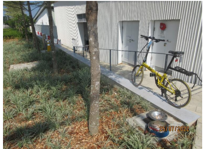
Some ties and stakes were removed along the Ting Kok Road.
