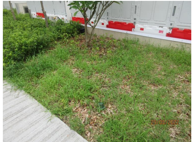
Some weeds were found in the planters along the Ting Kok Road.
