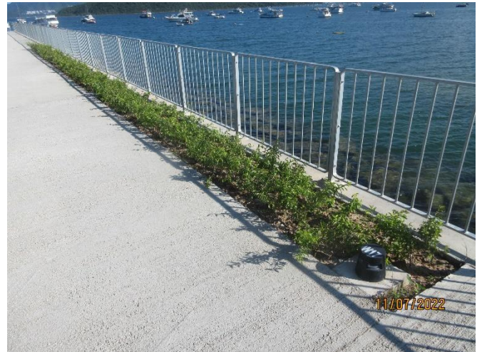
Plants in the planters on the Western groyne were replaced.
