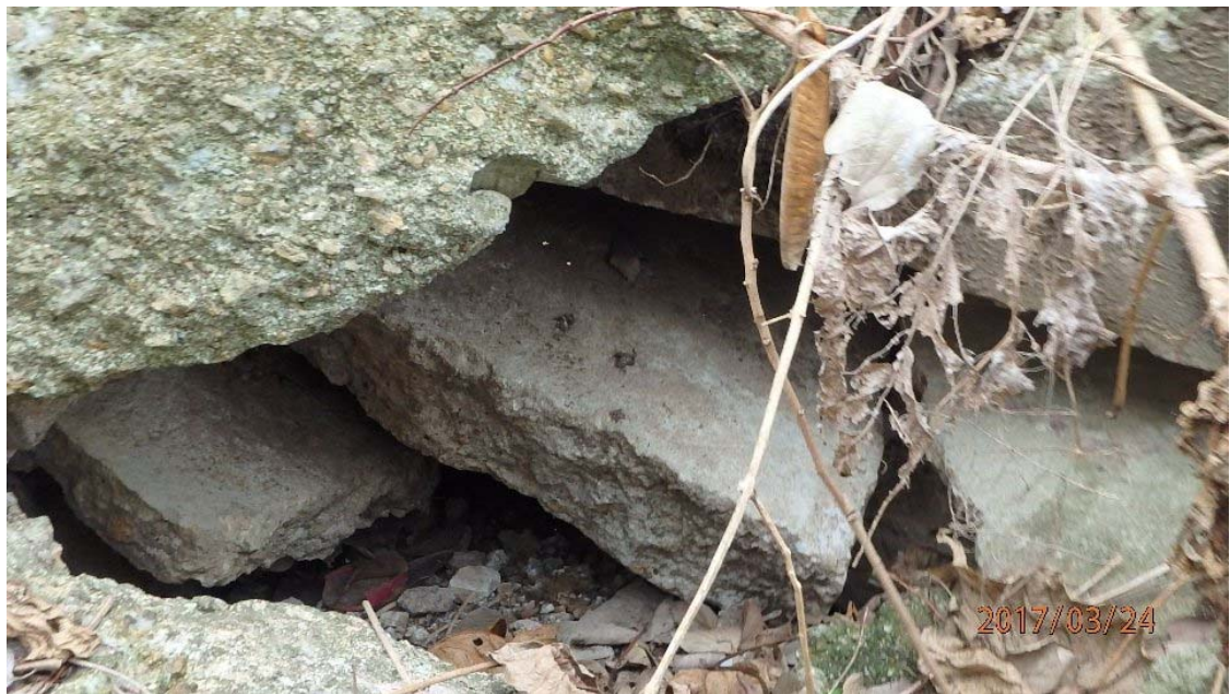
Photo 7. General View of Capture Survey Area
