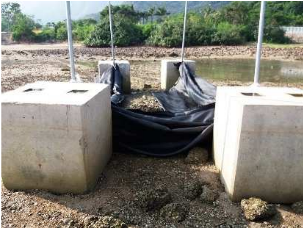
Photo 2. Demonstration of the fencing structure with concrete blocks and silt curtain on land
