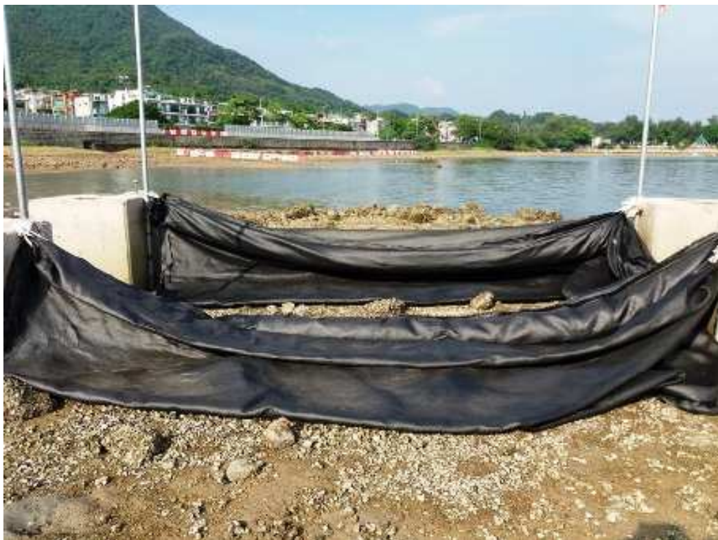
Photo 2. Demonstration of the fencing structure with concrete blocks and silt curtain on land
