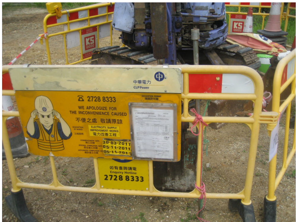
Photo 2 - One more plastic box folder for the environmental permit has been added.
