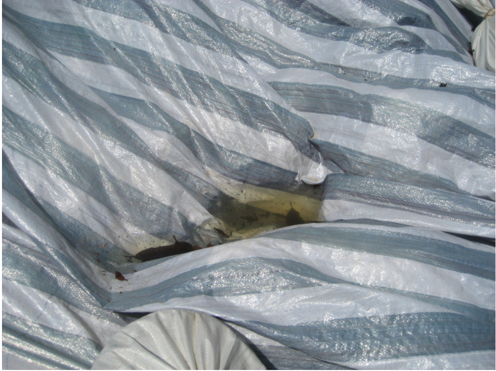
Photo 3 – Stagnant water was observed on the tarpaulin sheet covering the stockpile located next to the stream.
