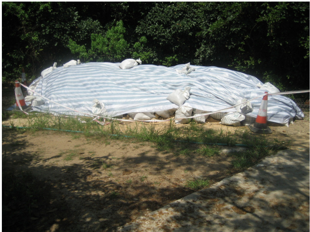
Photo 2 - Stockpile was observed adjacent to the stream.
