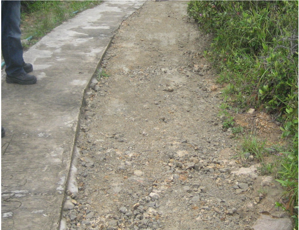
Photo 1 - The worksite for underground pipe and cabling works have been reinstated.
