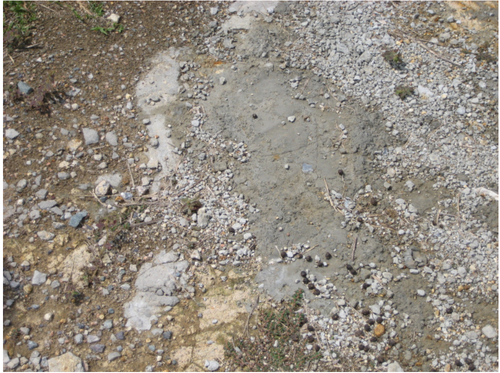
Photo 2 – Concrete stain near Site 1.
