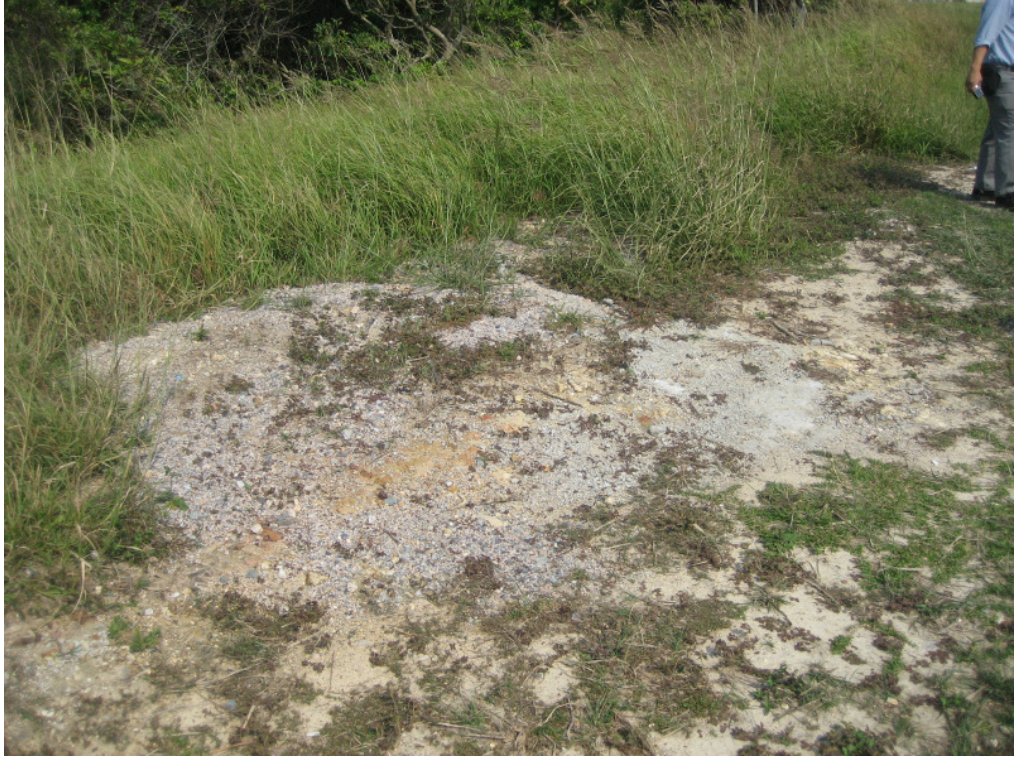
Photo 2 – The concrete stain on ground at Site 1 has been removed.
