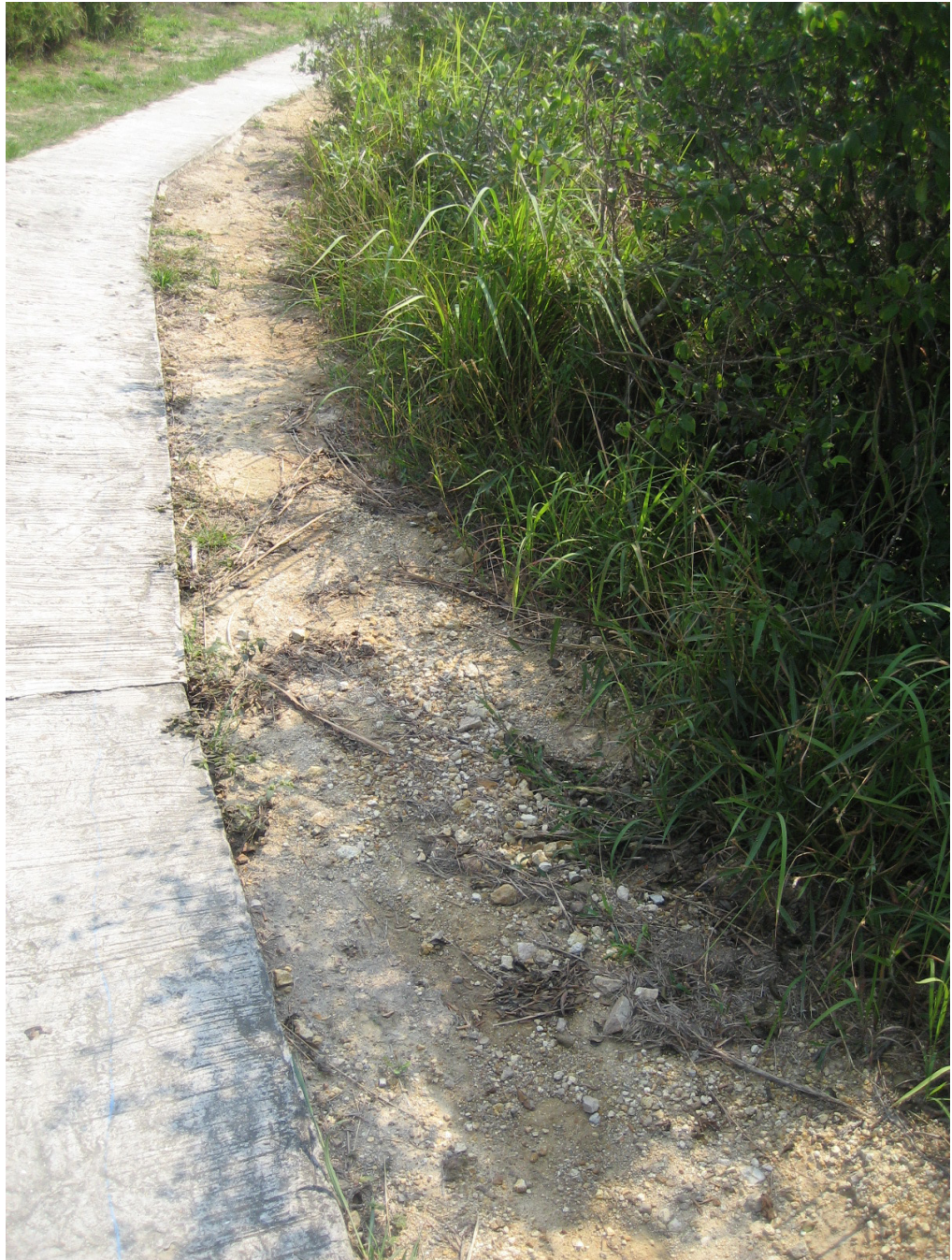
Photo 1 - The worksite for underground pipe and cabling works have been reinstated.
