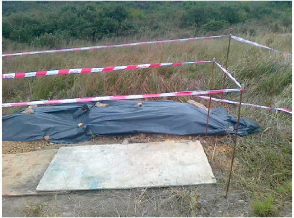
Photo 7 – The excavated material has been covered by impervious sheet.
