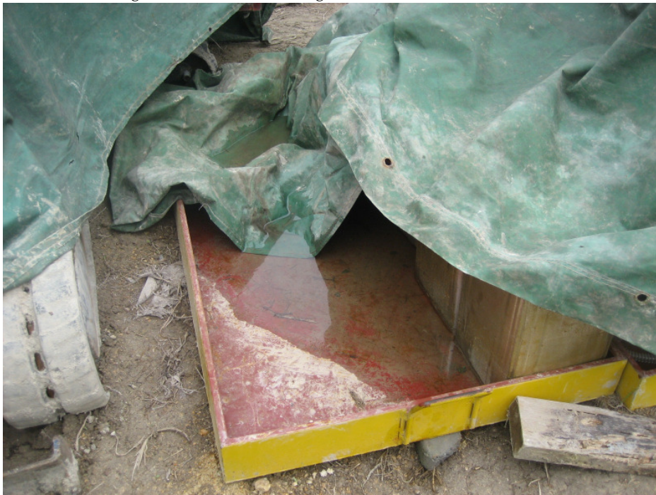
Photo 2 – Stagnant water was observed in drip traps at Site 1.
