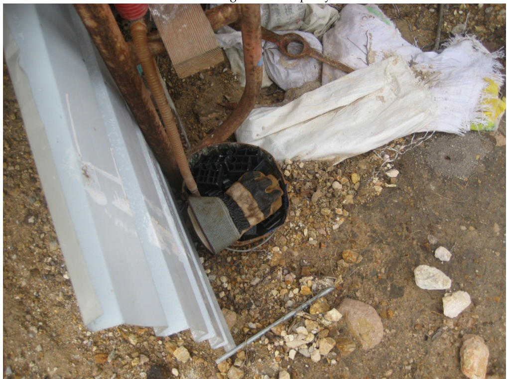
Photo 2 – Stagnant water was observed inside bucket and on tarpaulin sheet at Site 2.
