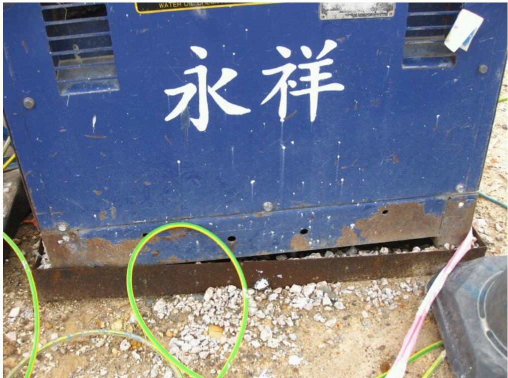
Photo 2 – The Contractor has plugged the hole immediately.
