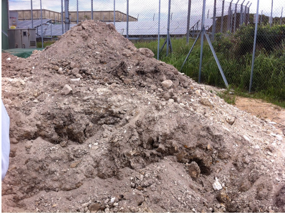
Photo 1 – Dusty stockpile was observed not being properly covered at Site 1.
