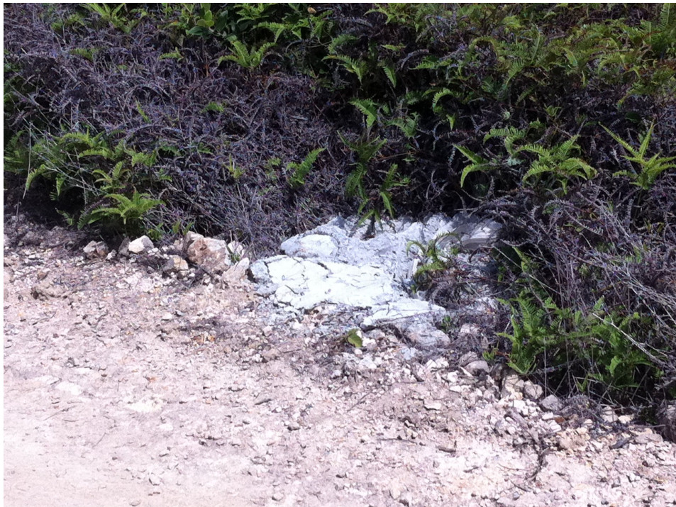
Photo 2 – Cement stain was observed outside the site boundary at Site 2.
