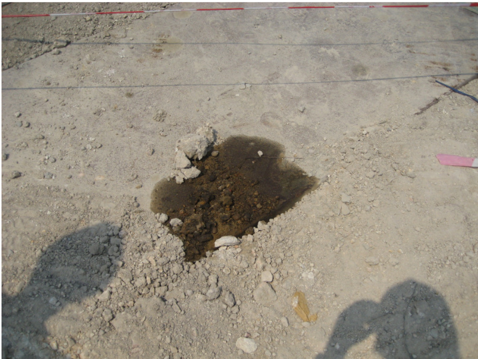
Photo 2 – Oil stain was observed on the ground after removing the generator
