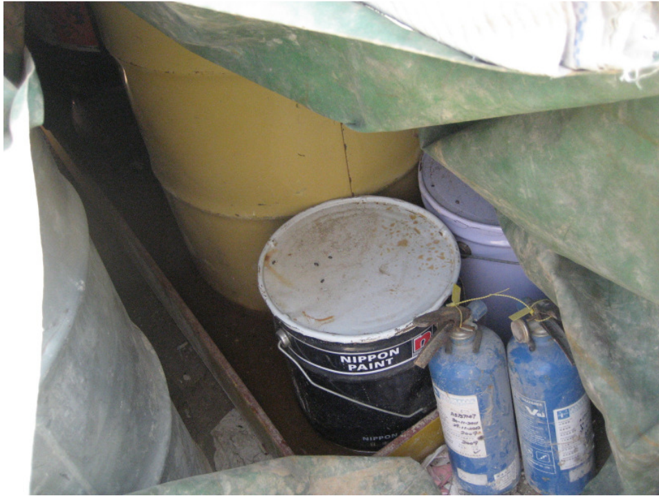
Photo 3 – Drip trays had been provided for the chemical drums at Site 1
