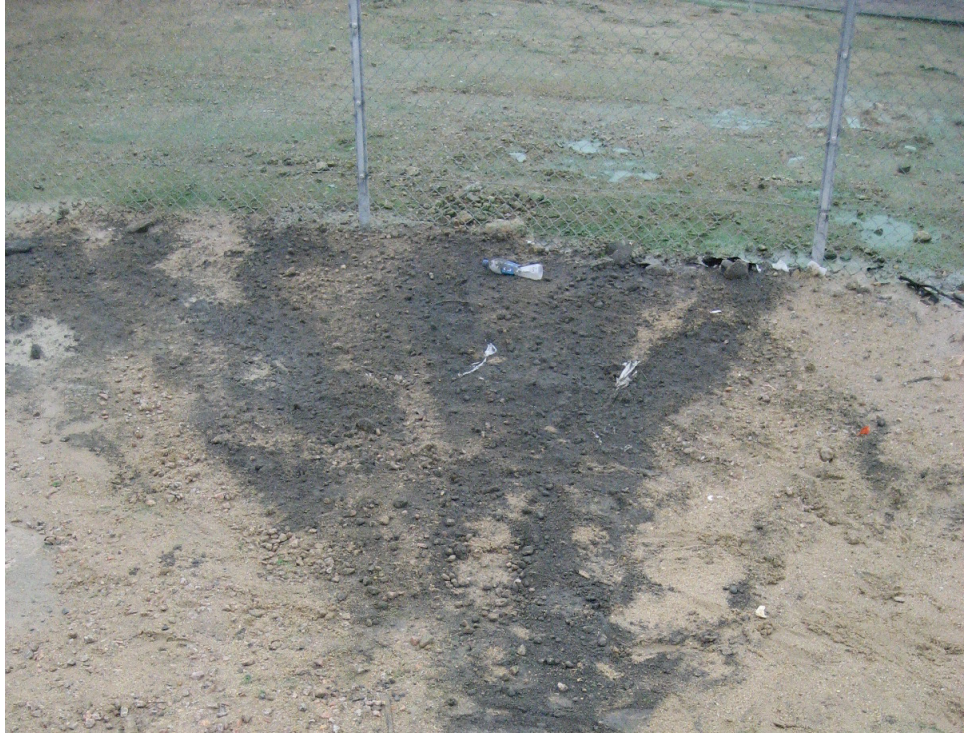
Photo 1 –Chemical stain was found on the ground near the entrance of Site 1.
