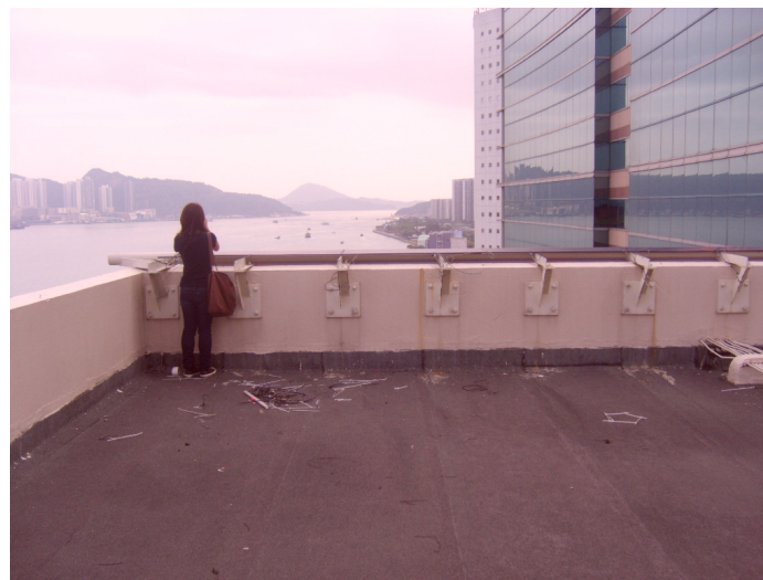
Monitoring location at FSQ
