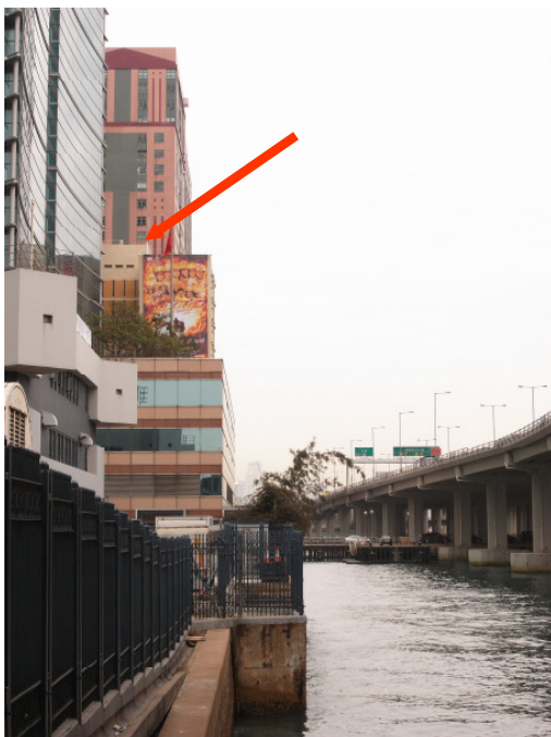
North Point Fire Services Married Quarters (FSQ)
