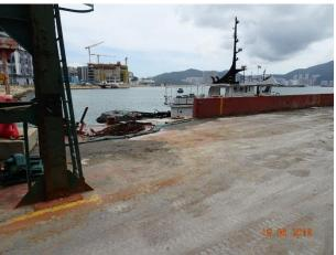
Sand bag was provided at working barge to avoid any runoff water leak into water body.
