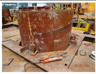
Cofferdam was used during marine bored pile work.
