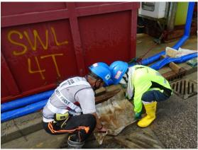
Geotextile was installed in the existing gully to prevent loose material flushing inside during rainstorm.
