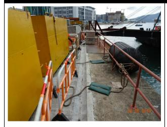
Cut-off drainage was installed at the site boundary to prevent muddy surface run-off leakage into the water body.
