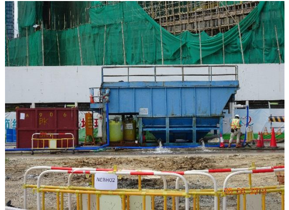
WetSept had been provided to treat any runoff water at Works Area A after the discharge licence is granted.
