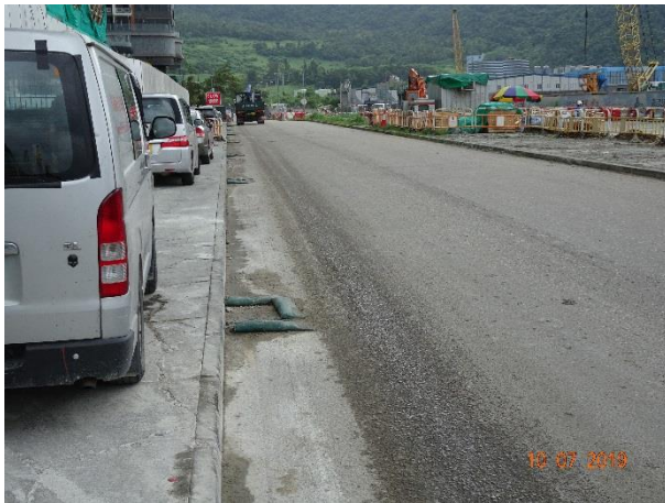
Sand bags had been provided for the existing manhole.
