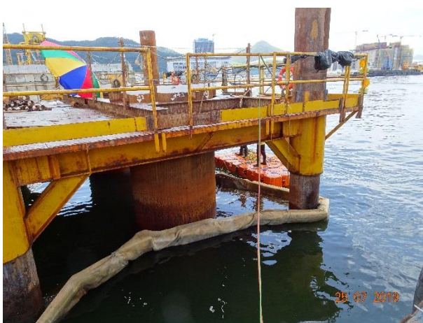
Silt-curtain had been provided for the piling platform.
