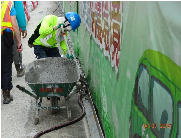
Gap between the concrete block and the sea front was sealed up.
