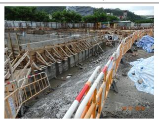
Concrete the exposed surface to reduce to create muddy water during rainstorm.
