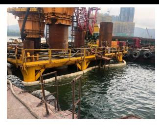
Silt curtain was installed to prevent the muddy water leakage into the water body.
