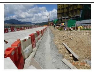
Part of the temporary drainage was installed to divert the site runoff to the de-silting facilities.
