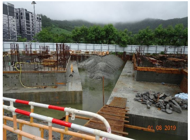
Exposed slope had been shotcrete to reduce generated of turbidity water.
