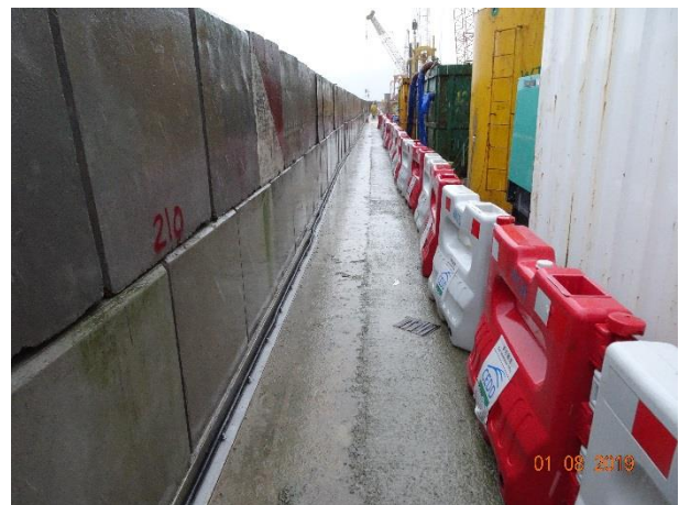
Gap between the concrete block and the sea front was sealed up.
