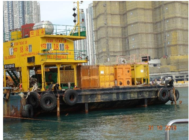
De-silting facilities had been provided to treat the site generated water prior discharge.
