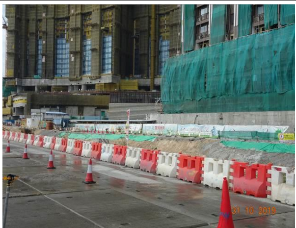
Using tarpaulin cover the exposed area to prevent generate turbidity runoff during rainstorm.
