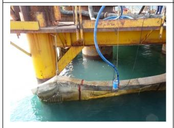
Silt-curtain had beed provided to prevent muddy water overflow from the piling platform.
