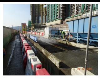
Treatment facilities was installed at site to treat the site generated water prior discharge.
