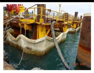
Silt-curtain had beed provided to prevent muddy water overflow from the piling platform.
