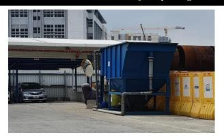
Treatment facilities was installed at site to treat the site generated water prior discharge.
